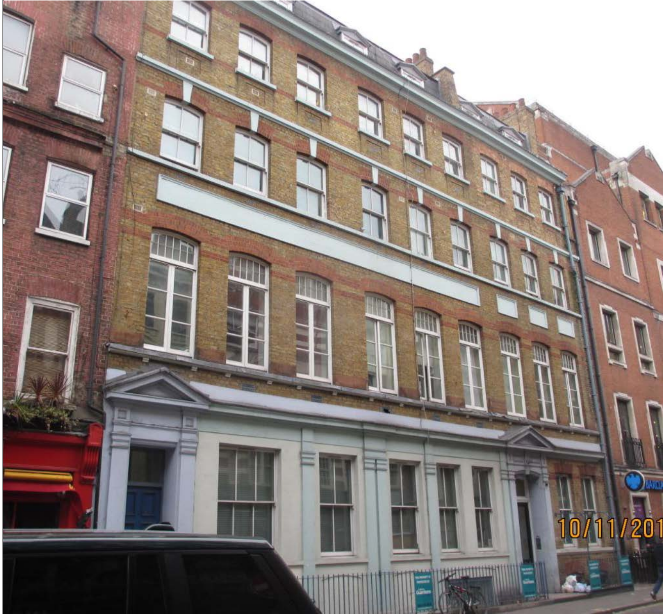
The site prior to conversion of the upper floors
