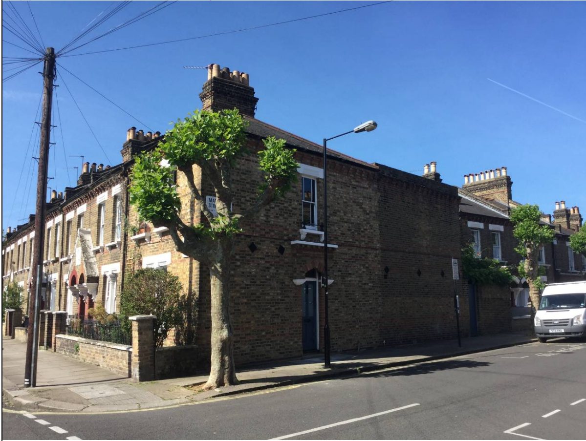
Application Site viewed from junction with Marne Street
