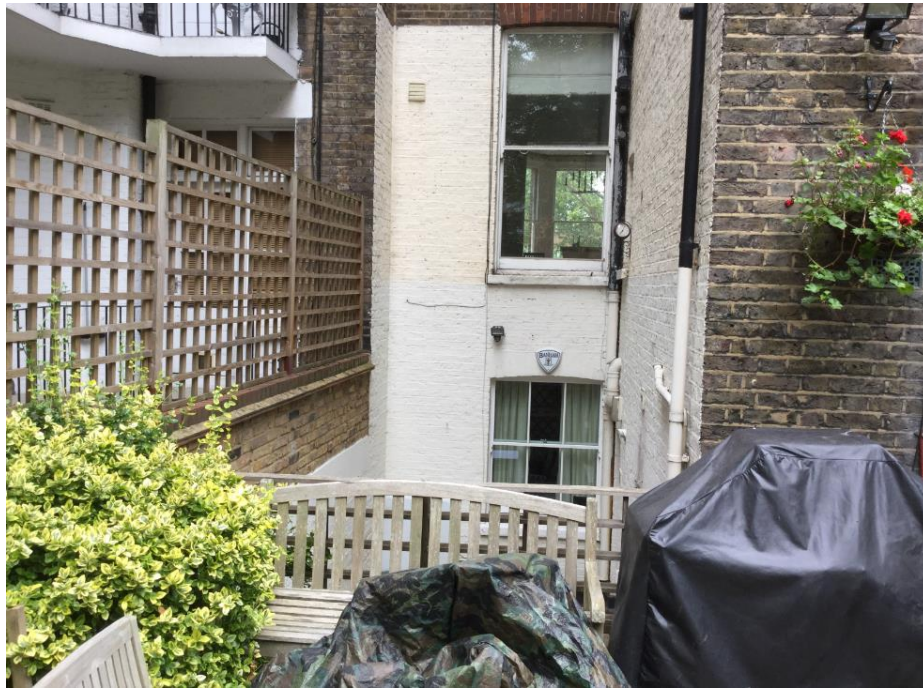
View of Infill Extension Location
