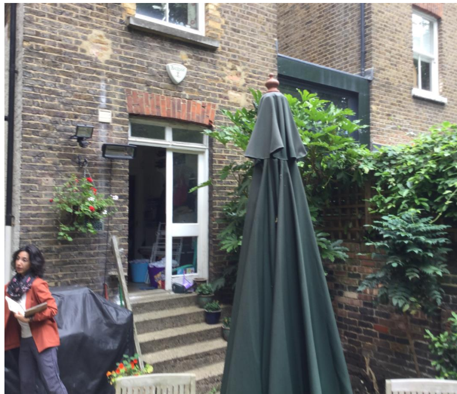
Rear of Existing Closet Wing
